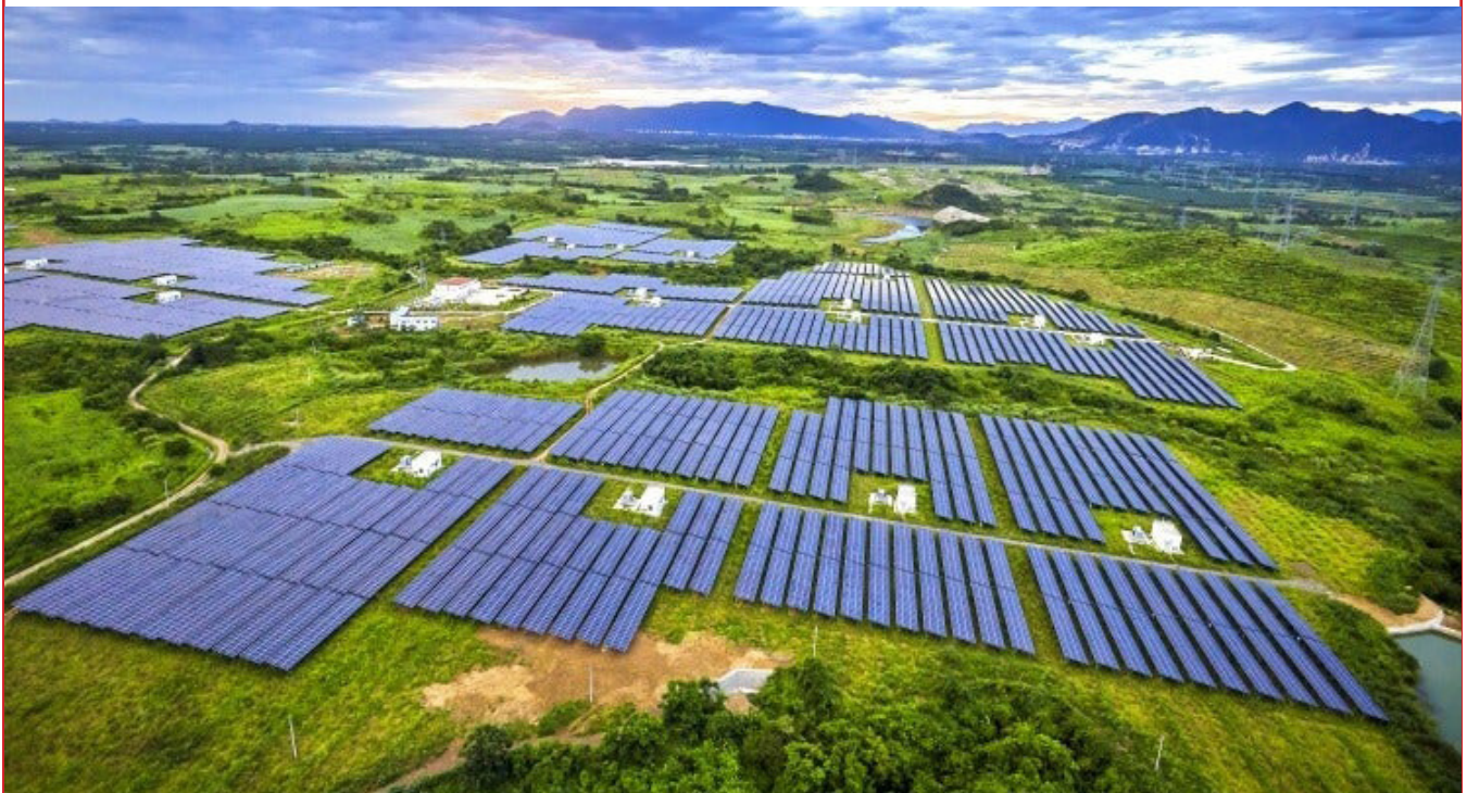
Figure 1 - Aerial View of Inverters and Transformers Located Throughout a Solar Facility (2025) DNV.com
